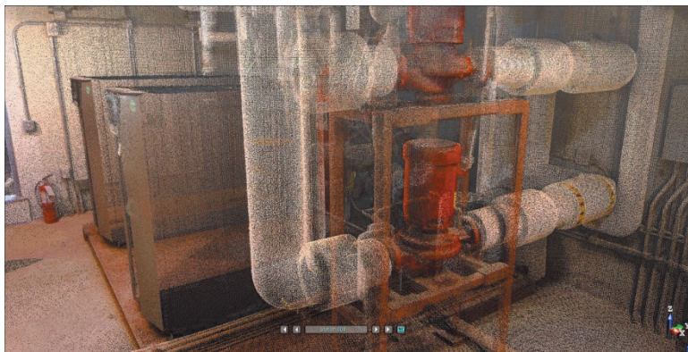
Figure 7: Colorized point cloud in RealWorks Station Based view
